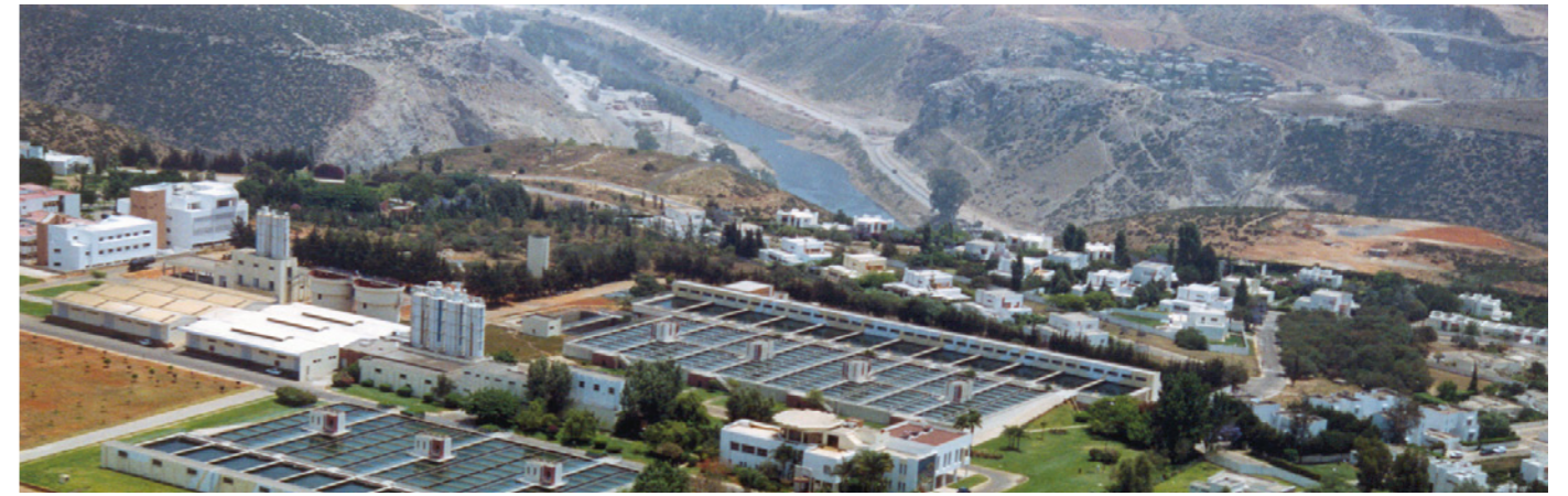
Bouregreg water treatment station of ONEP in Rabat, Morocco.
