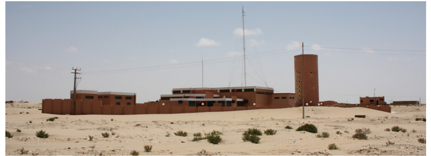
Desalination plant on the Saharan coastline, Tarfaya, 2010.
