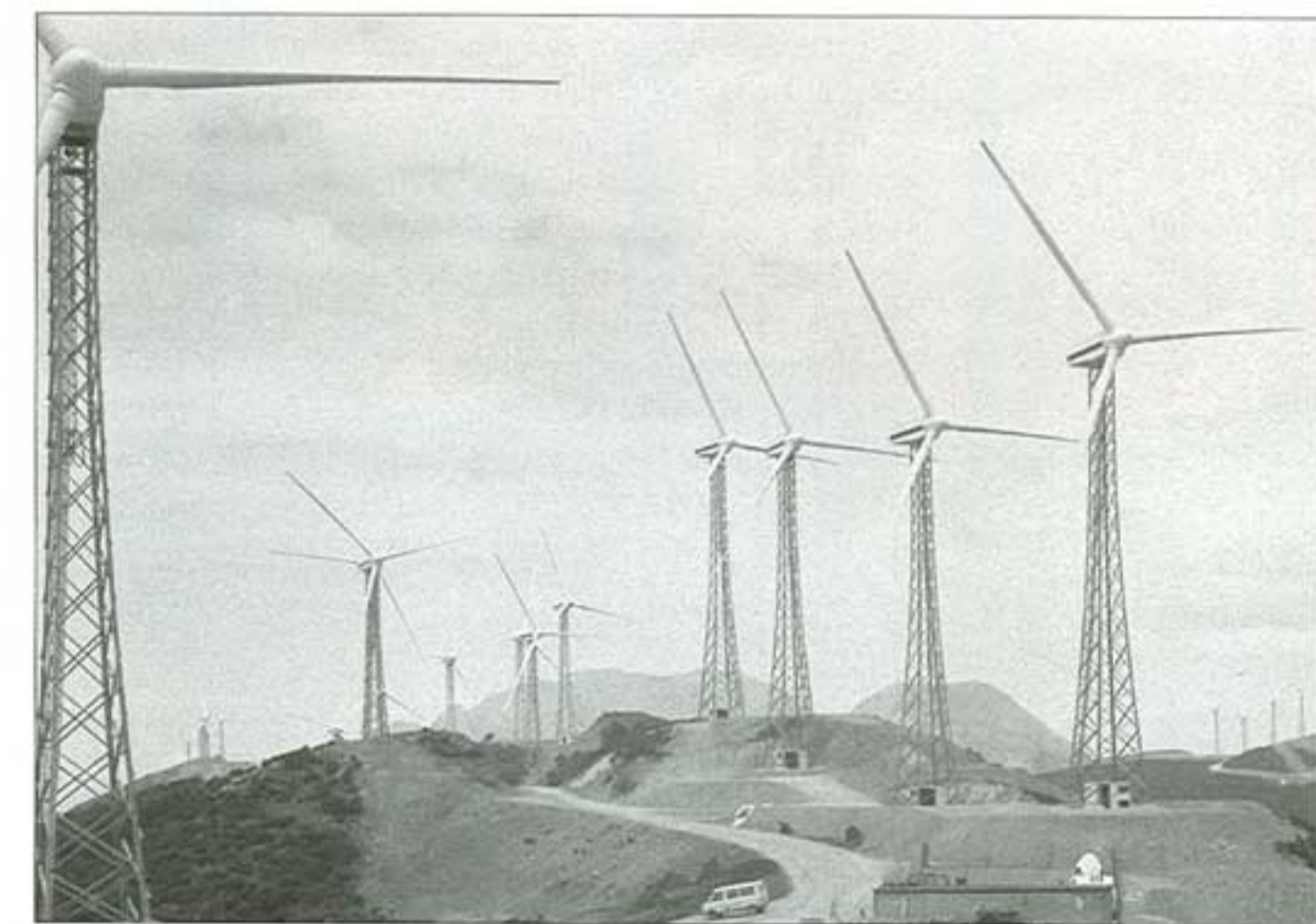
Potential: The 50 MW farm at Al Koudia al Baida is Morocco's only large scale wind power station, though if all goes well national capacity will soon be boosted by 200 MW
